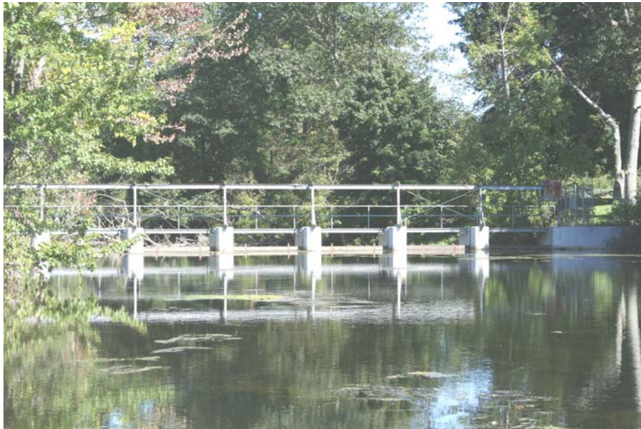
Winnie's Reef - Stop Log Structure.
