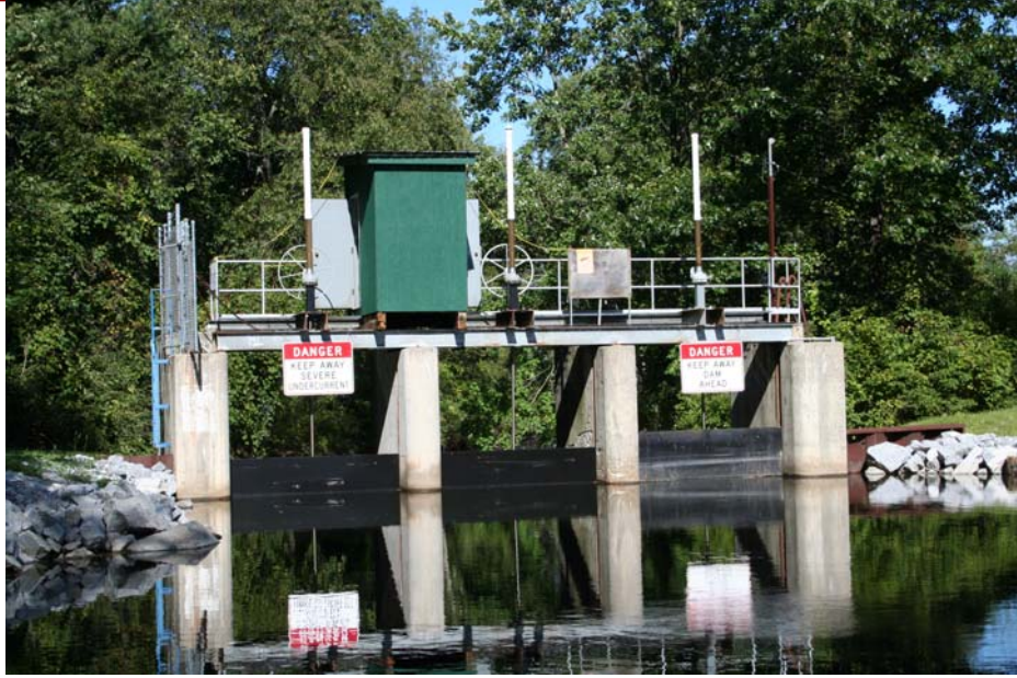
Winnie's Reef - Sluice Gate Structure.
